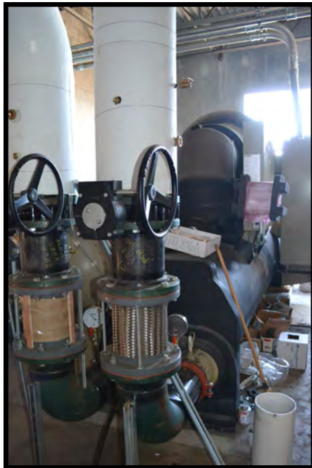
(LEFT) This 450-ton chiller has been installed next to a smaller 250-ton unit. The butterfly valves are from Stockham, the flexible connectors are from Flex-Hose, and the thermometers are from Terrice.
