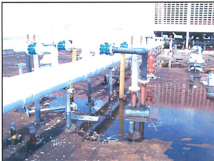
(ABOVE) A view from the rooftop where the copper tube risers terminate. The risers, 17' 4" tubes from Cerro Flow Products, were cut in half and grooved at the A&B fabrication shop, a handling facilitation required on each floor of the building. The chill water return is collected in a 16" PVC schedule 80 pipe and fed into the top of the new cooling tower shown in the background. The PVC replaced the original steel pipe.
