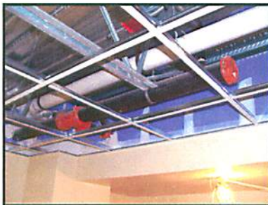
(LEFT) The view from the end luxury suite, highlighting the main sprinkler pipe with Victaulic Firelock fittings.
